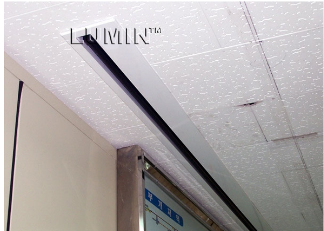
Recessed Ceiling installation
